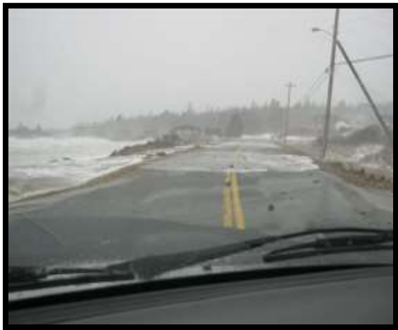
Locke Street West during storm surge Feb 2013
