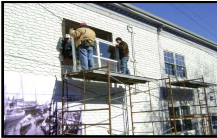
Energy efficient windows being installed at the Town Office building winter 2013.
