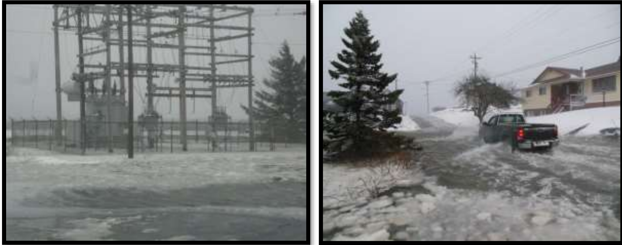
Storm surge at intersection of North and Upper Water Streets, Feb. 2013, 16 inches of water and ice.
